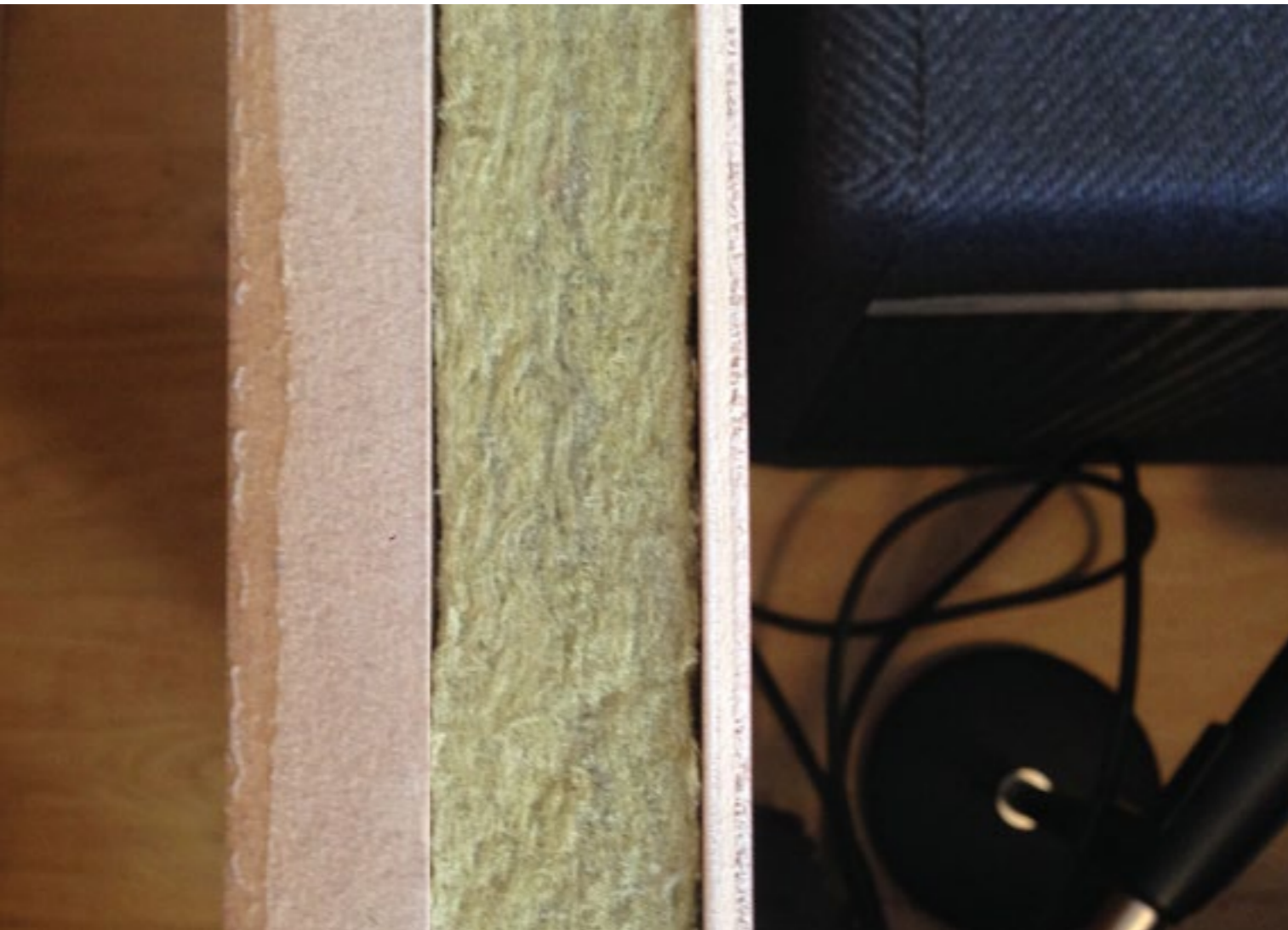
A view from the top showing the three layers of the left hand panel - from right to left; 18mm (MDF shell) + 30mm (rock wool layer) + 5mm (plywood layer)
